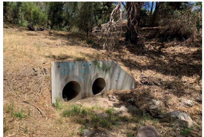
Figure 12. Downstream outlet detention basin.
