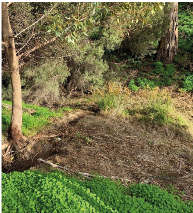
Figure 6. Erosion caused by stormwater flows.
