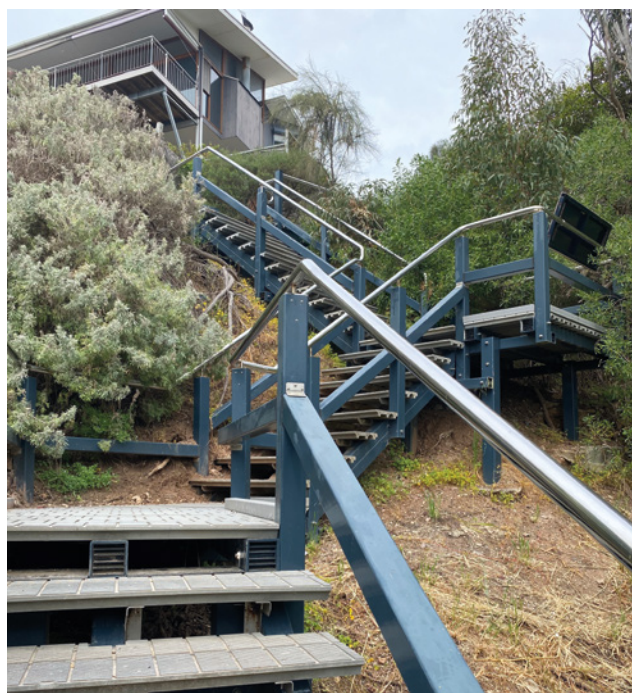
Figure 2. Composite fibre and recycled plastic staircase.
