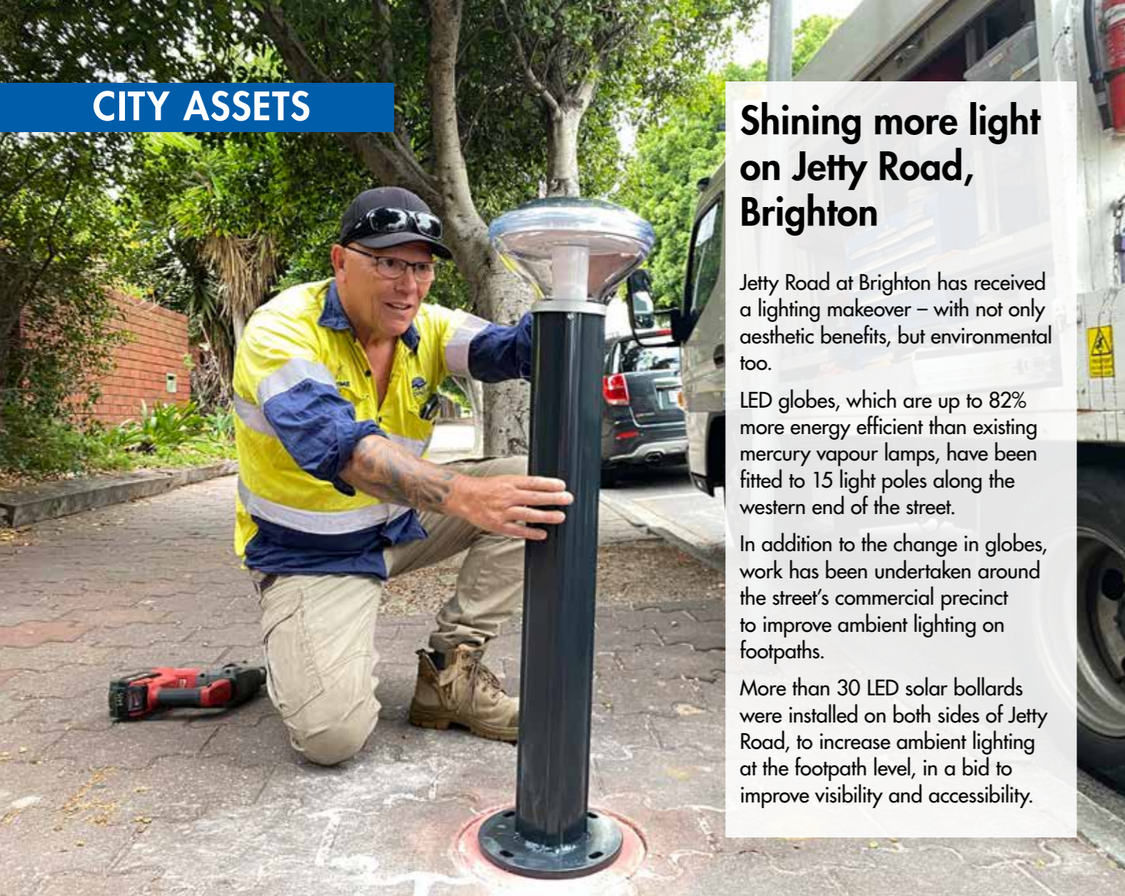
Dene from Council's Field Services team installing one of 30 solar bollards on Jetty Road, Brighton.
