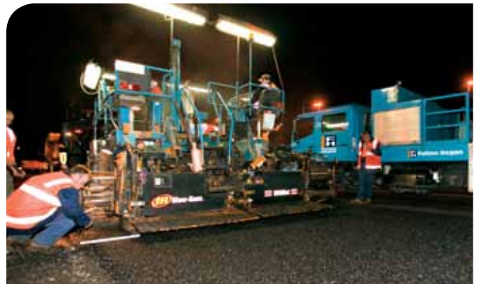
Research indicates that Warm Mix Asphalt is equally as effective in creating asphalt pavements as Hot Mix Asphalt and boasts additional environmental benefits and increased safety for crews handling the asphalt.
