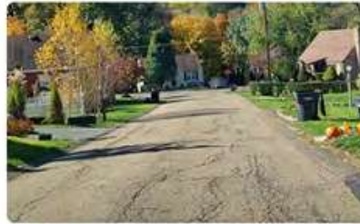
Fatigue Cracking
