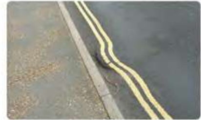
Pavement Distortions
