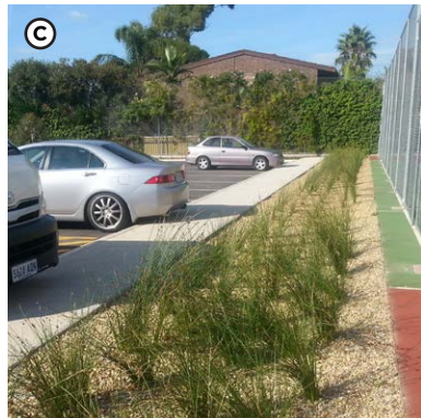
C WSUD Rocky Swale to capture storm water run-off from new car park
