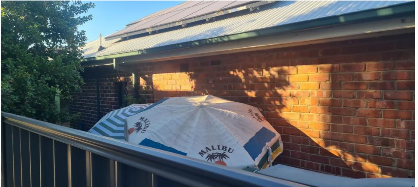
Figure 2: View of Side Yard of 6 Goldsworthy Crescent Adjacent the Alfresco Wall of 8 Goldsworthy Crescent
