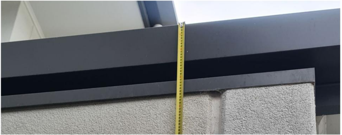
Figure 3: Typical Boundary Gutter Detail
