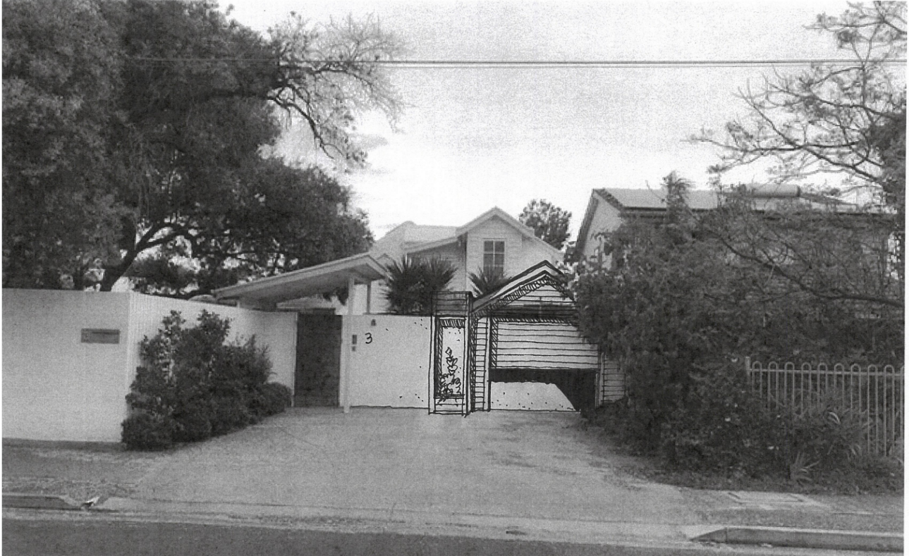
Figure 2: Streetscape view of the subject site with carport superimposed
