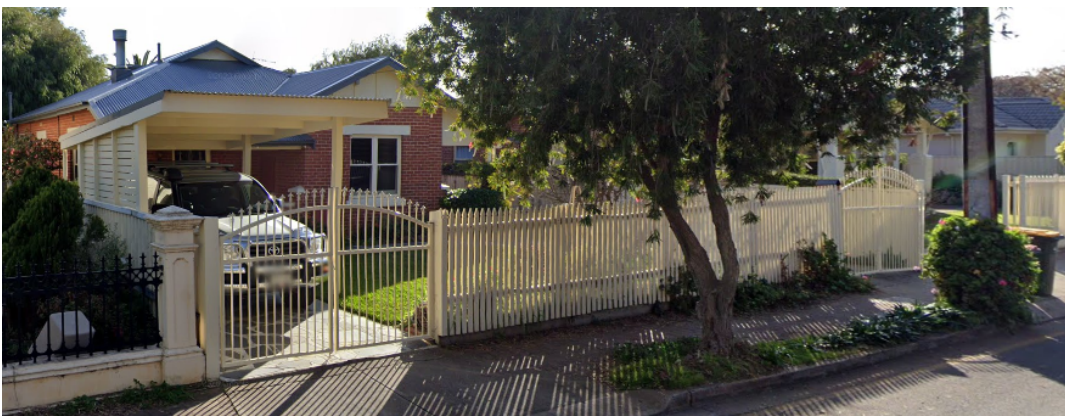
Figure 3: Carport located forward of dwelling located at 10 Dunluce Avenue
