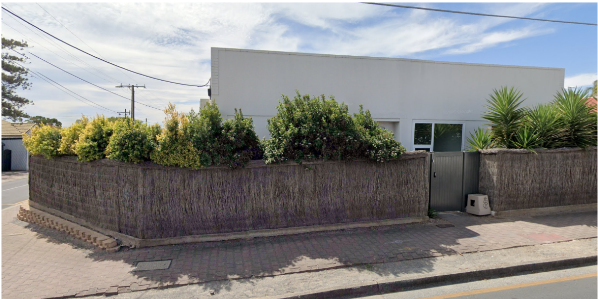
54 Wheatland Street - North-eastern corner
