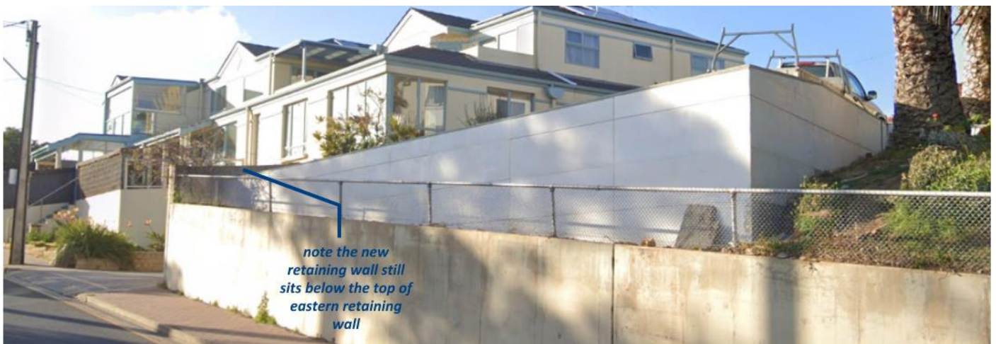
August 2020 Google Street View showing new retaining wall facilitating a flat base.
