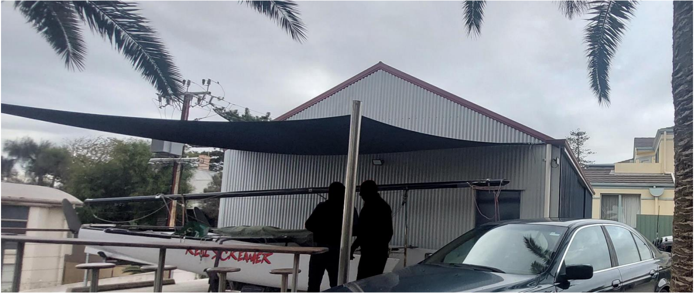
The shed is clad with corrugated iron sheeting and has a 25 degree pitch
