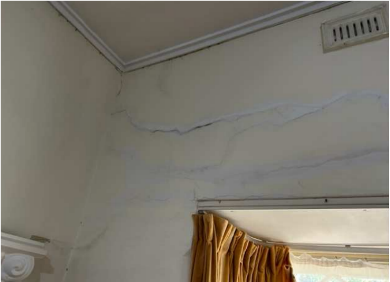
Photo showing cracking inside the dwelling
