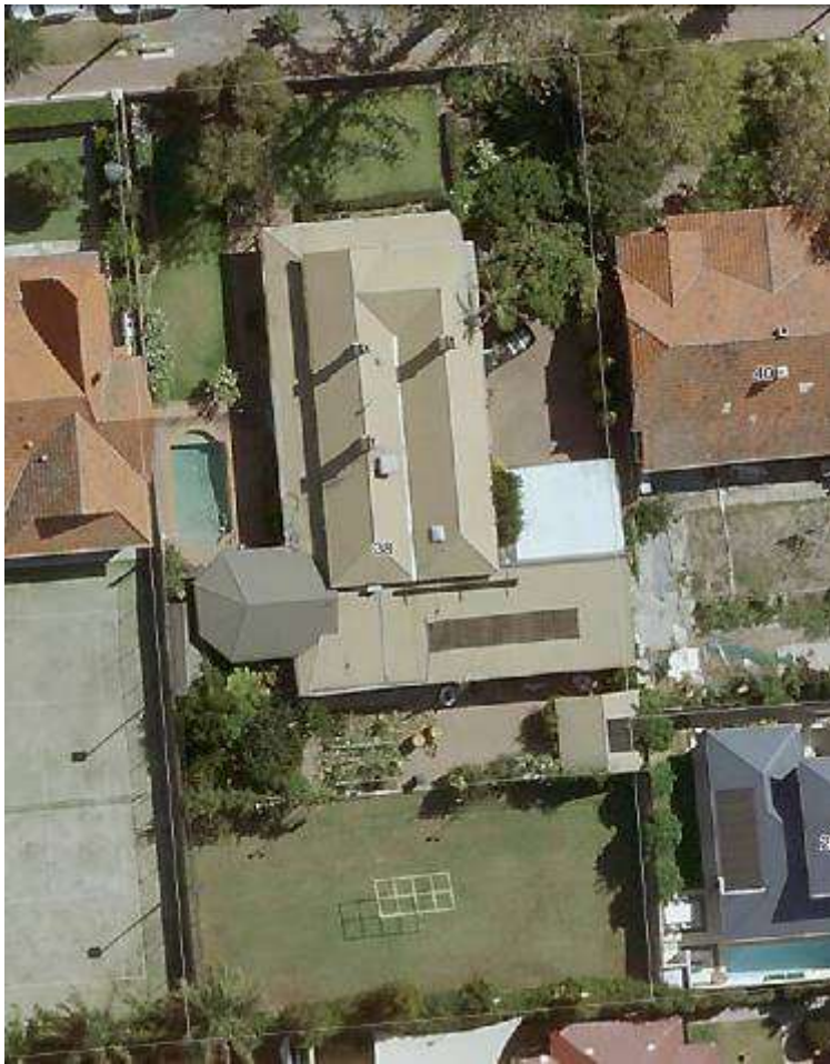
Aerial view of the property at 38 Broadway
