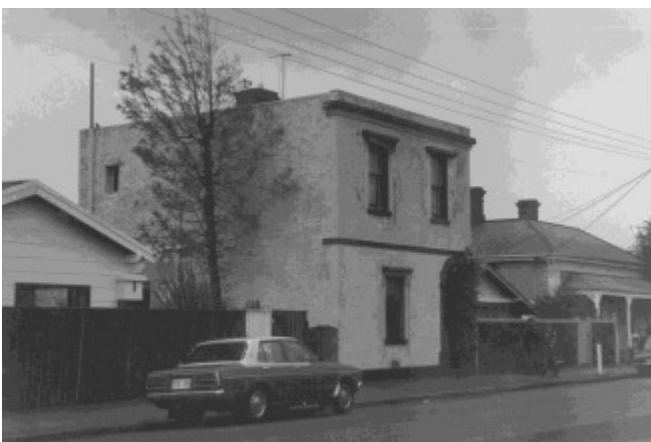
34 Waterloo Street, 1980 - PH-GL-1183 Holdfast Bay History Collection
