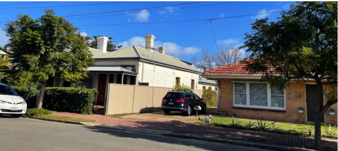
3D render prepared by Dash Architects to demonstrate the appearance from the streetscape
