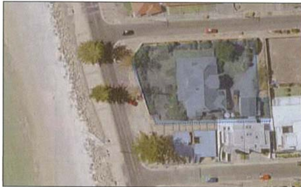
Aerial view of the subject property showing approximate site boundary of Lot 15 (highlighted blue) and extent of improvements over the site
