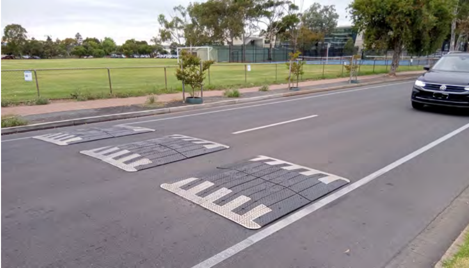
Figure 2. Speed cushion arrangement on King George Avenue
