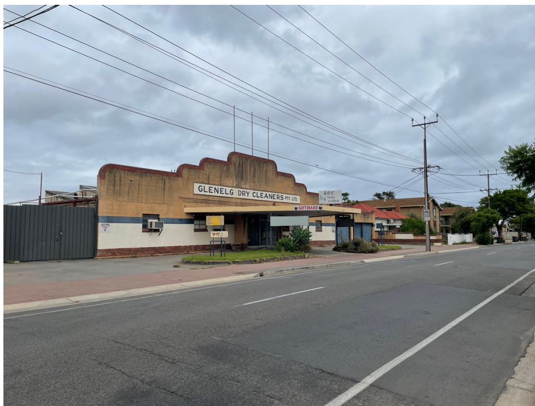
37-41 Cliff Street view from the East
