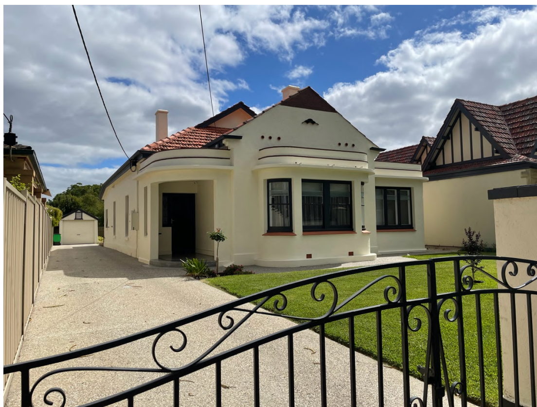
View of 25 Broadway from the south.
