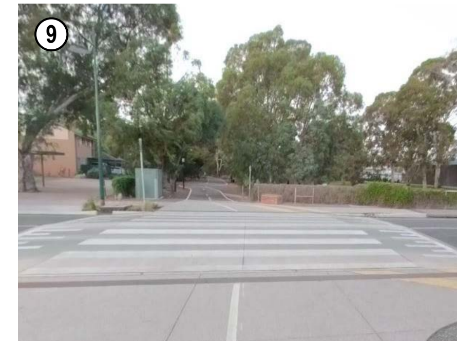
9 - Raised pedestrian crossing
