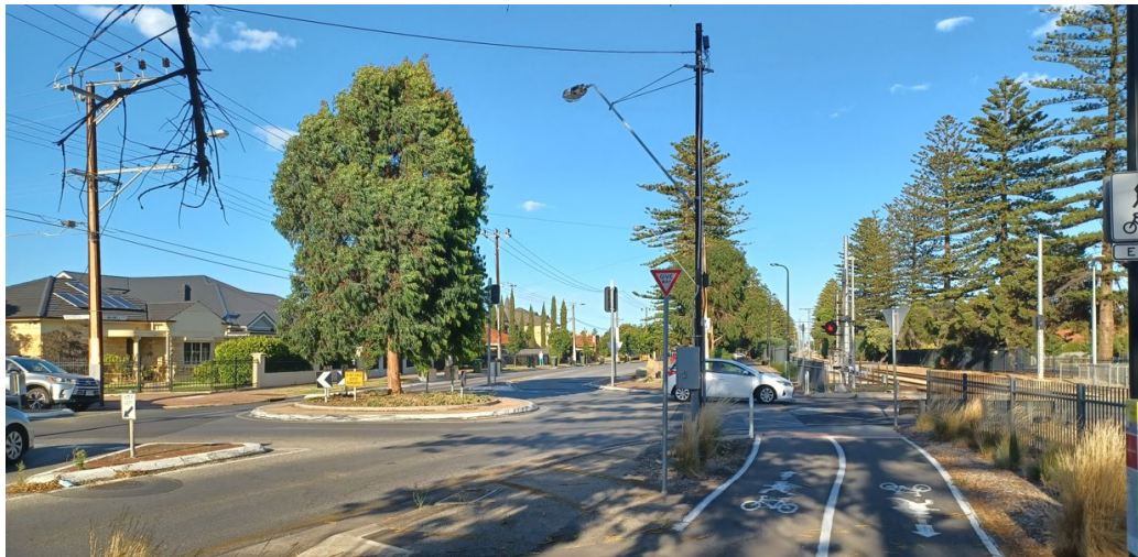
Car queuing on roundabout – Had already entered roundabout before boom gates activated
