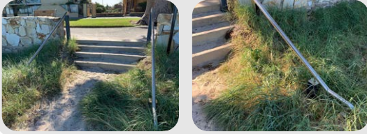
Site 3 - Stairway being surrounded with sand & vegetation
