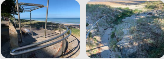
Site 2 - Timber Decking with ramp buried in sand
