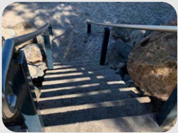
Site 5 - Stairway with lower end buried in sand
