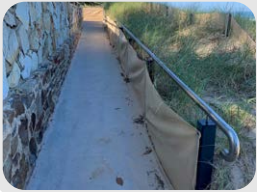
Site 4 - High maintenance ramp between wall and sand dune
