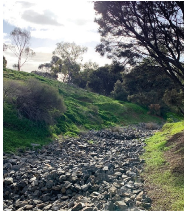
Figure 7. Excessive watercourse rock lining.
