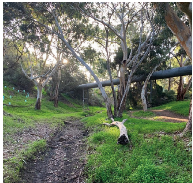
Figure 15. Water supply crossing.
