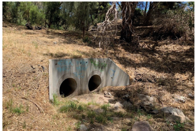
Figure 12. Downstream outlet detention basin.
