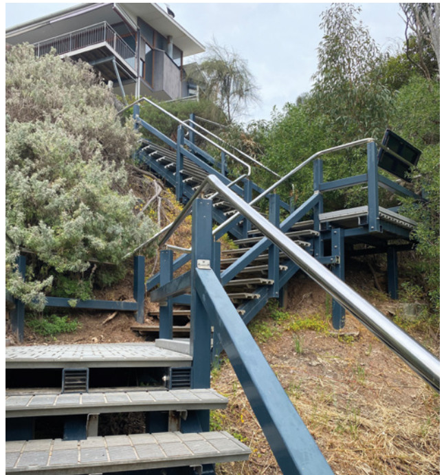
Figure 2. Composite fibre and recycled plastic staircase.
