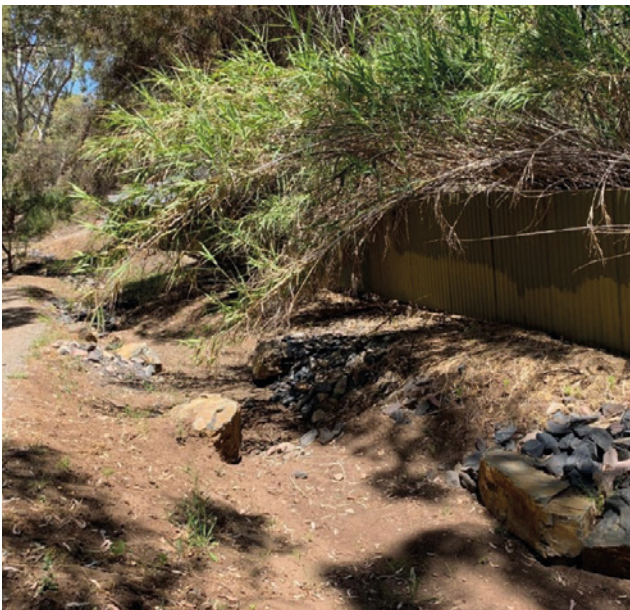
Figure 14. Erosion along drainage line.
