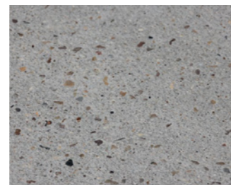
06 In-Situ Concrete Lightly washed exposed aggregate concrete
