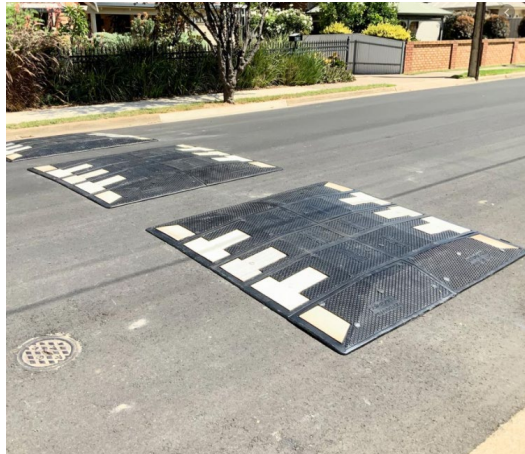
Example of road cushions
