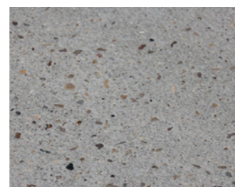
06 In-Situ Concrete Lightly washed exposed aggregate concrete
