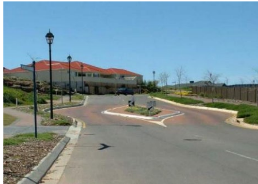
Example of centre blister island
