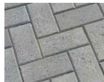
03 Pre-Cast Concrete Paver Pre-cast concrete - Adbri Havenbrick
