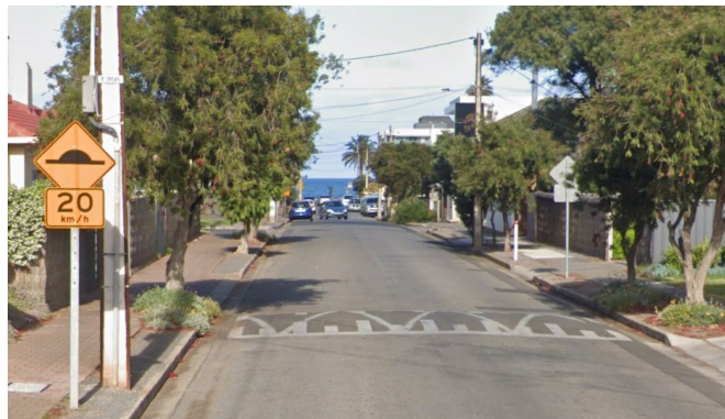
Example of road humps
