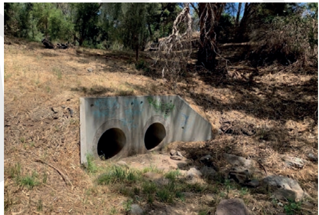
Figure 12. Downstream outlet detention basin.
