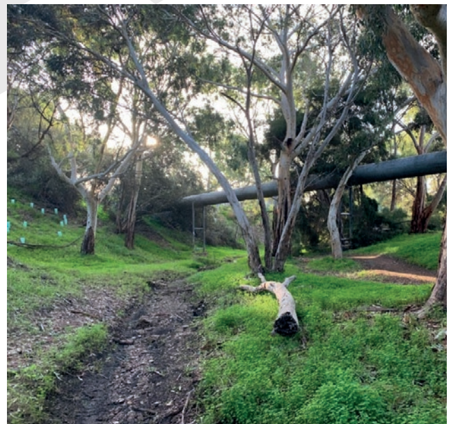
Figure 15. Water supply crossing.
