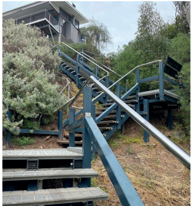
Figure 2. Composite fibre and recycled plastic staircase.
