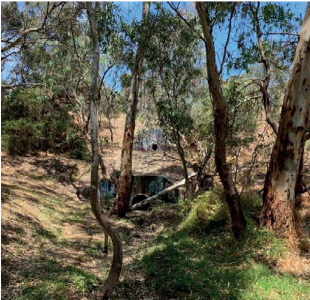
Figure 11. Upstream drainage infrastructure.
