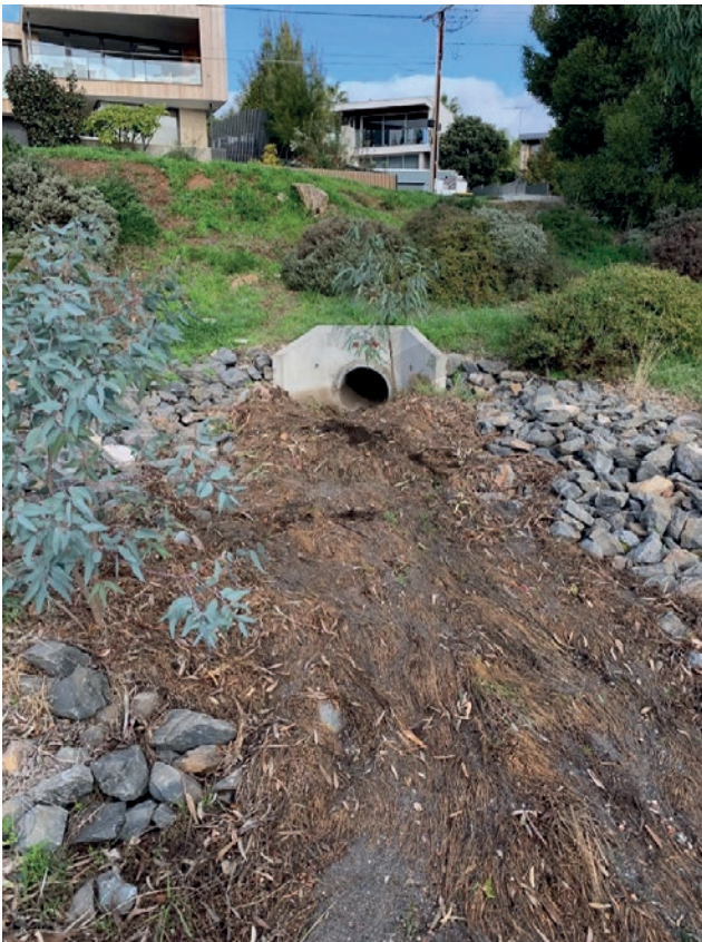
Figure 12. Barton Road stormwater discharge into Barton Gully.
