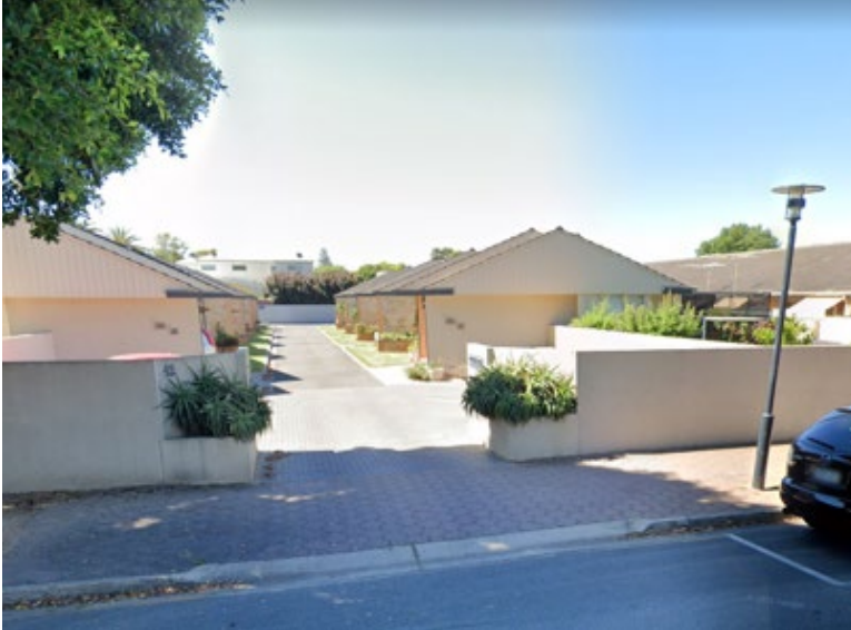
Figure 2: 42 Jetty Road driveway access
