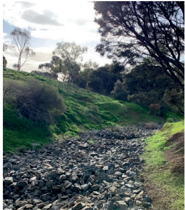
Figure 7. Excessive watercourse rock lining.
