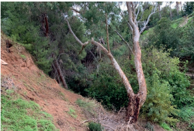
Figure 10. Downstream of upstream outfall.
