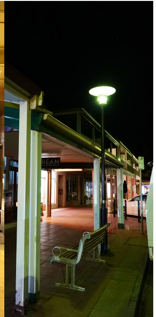
Existing pedestrian lighting outside of C.R.E.A.M has minimal impact as the majority of light output is obstructed by the protruding verandah.
