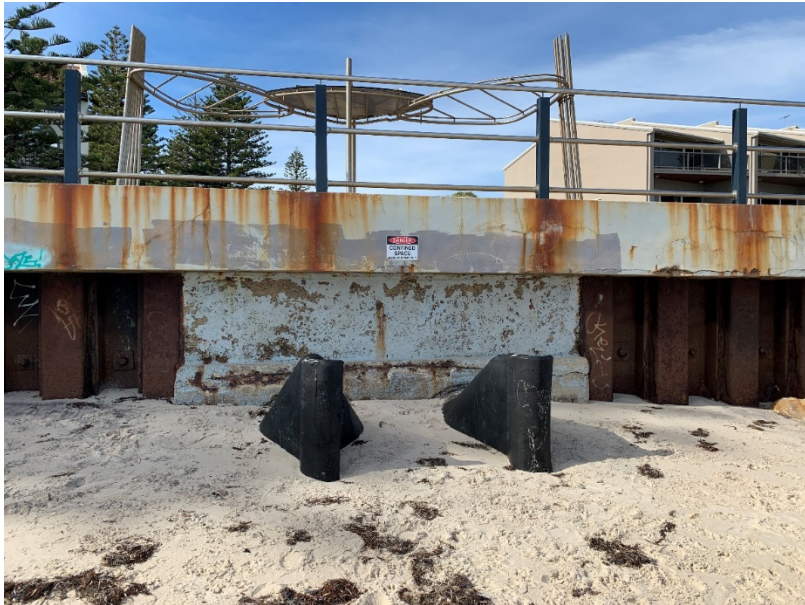
Photo 2 Pier Street outfalls
