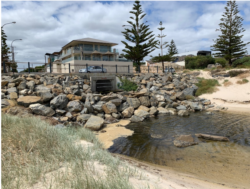
Photo 4 – SWSDS Outlet – Edward Street – polluted ponding water
