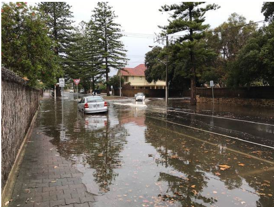
Pier Street Glenelg – local flooding
