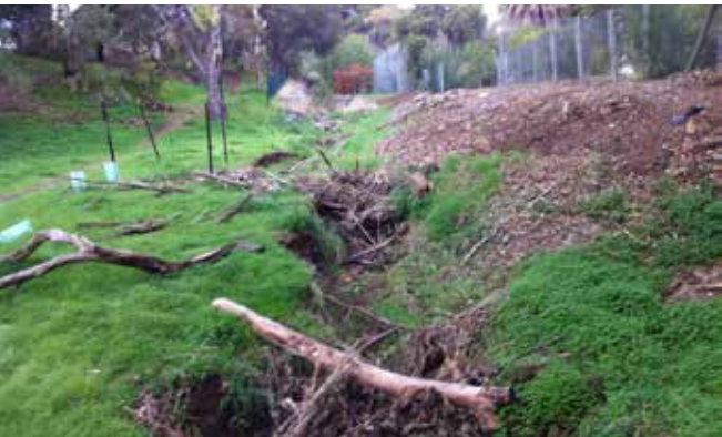
Debris within the watercourse causing blockages
