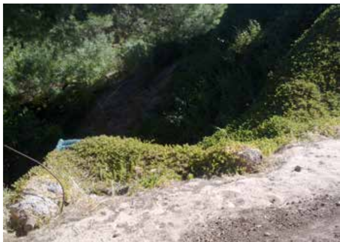
Steep drop-off into gully to be rectified with pipe extension and drop pits
