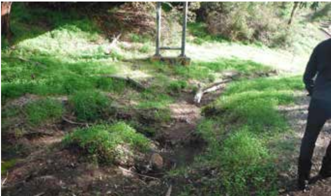
Erosion (underneath water supply crossing)
