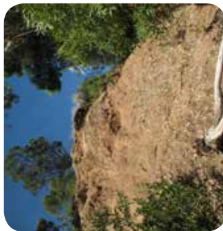
Eroded embankment
