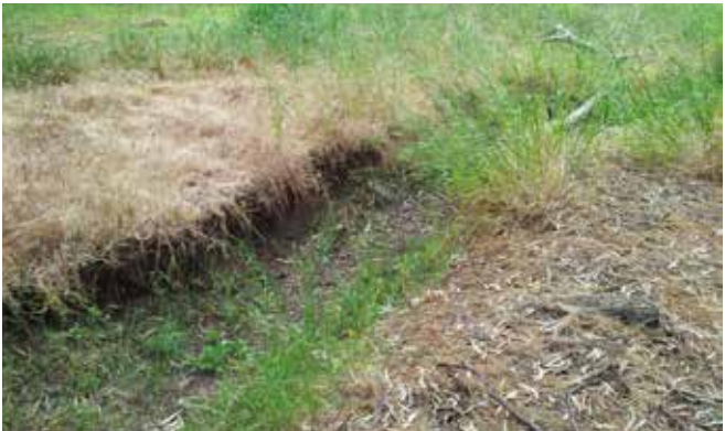
Erosion along the main drainage line
