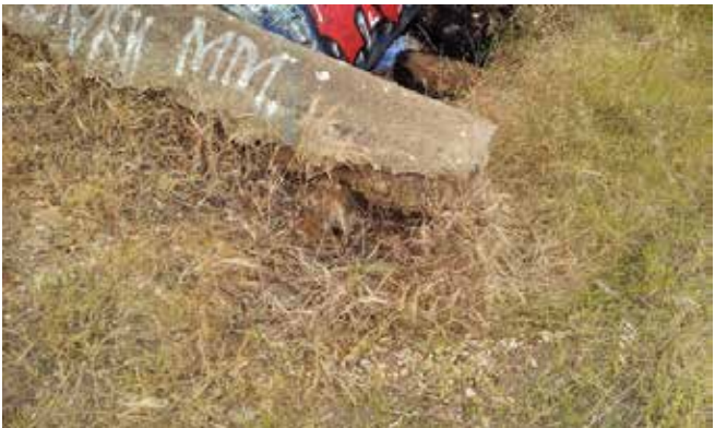
Damage and erosion at SA Water pipe headwall
