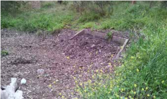
Detention basin culvert trash screen
