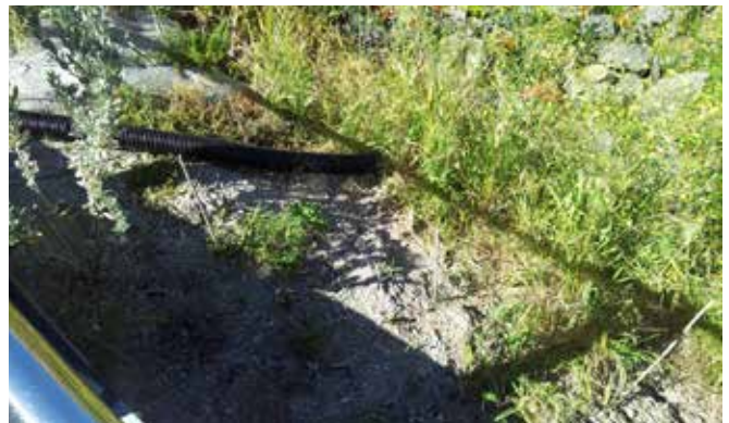
Existing pipe redirecting stormwater flows
