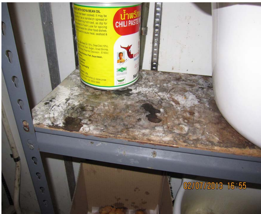
Figure 6: Shelf in the cold room, fabricated from untreated particle board – unable to be effectively cleaned and contaminated by mould.
