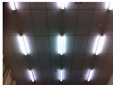
Figure 1 Stage 2 of Civic Centre Lighting Upgrade
