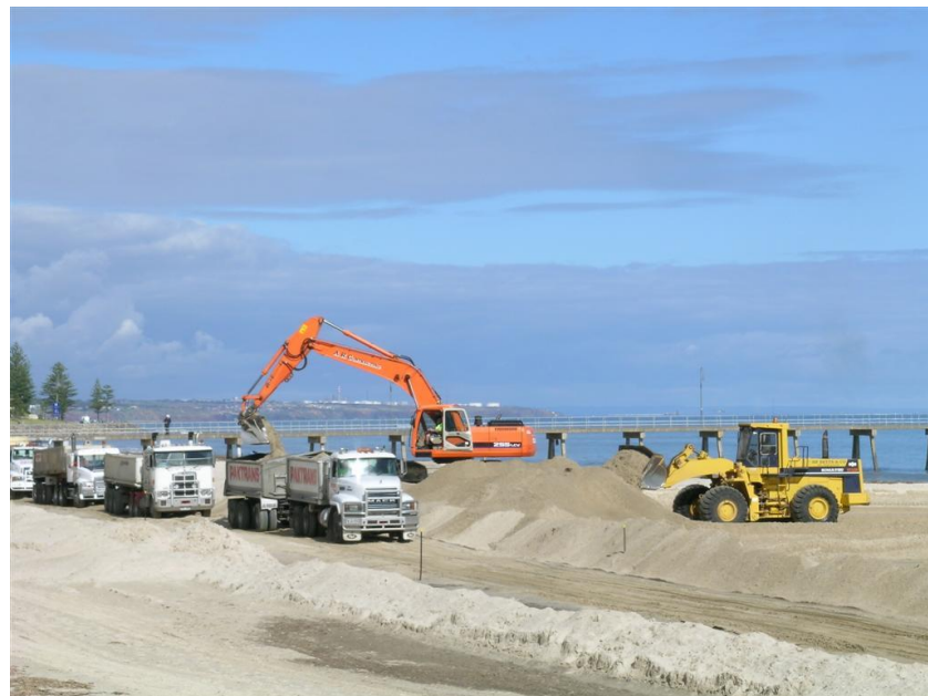
Sand carting trucks in use at Glenelg Jetty (this method of operation is being superseded here).
