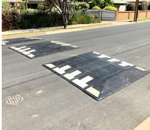
Example of road cushions
