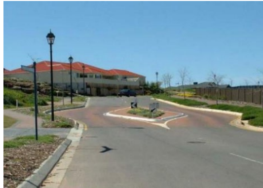
Example of centre blister island
